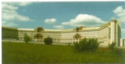
The New Building of the Bakoulev Institute.
